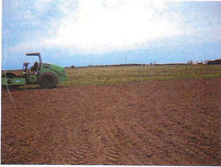
View South Project site located behind heavy equipment
