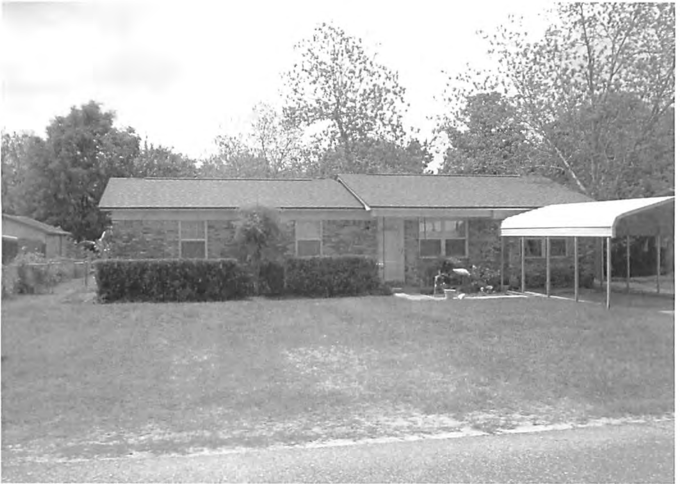
Electrical Wiring upgrade 1005 Colbert Avenue
