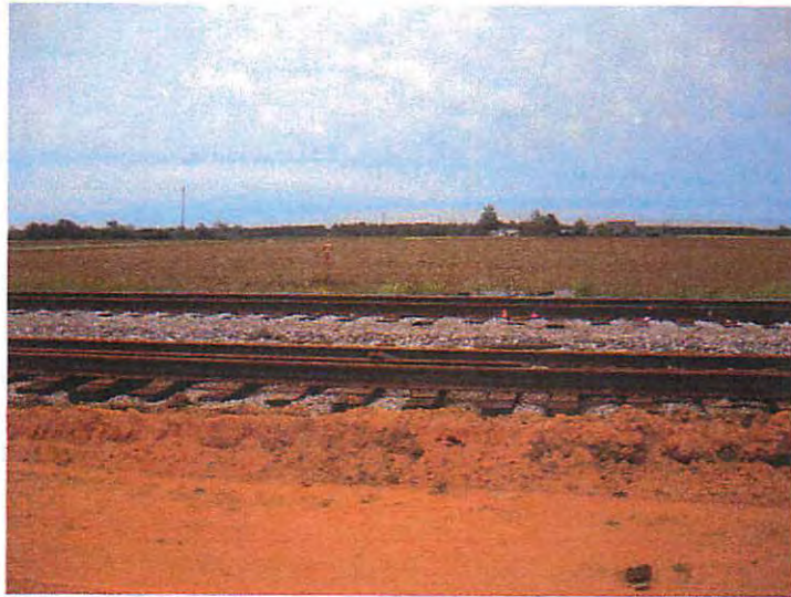
Existing railway, and pipeline monument
