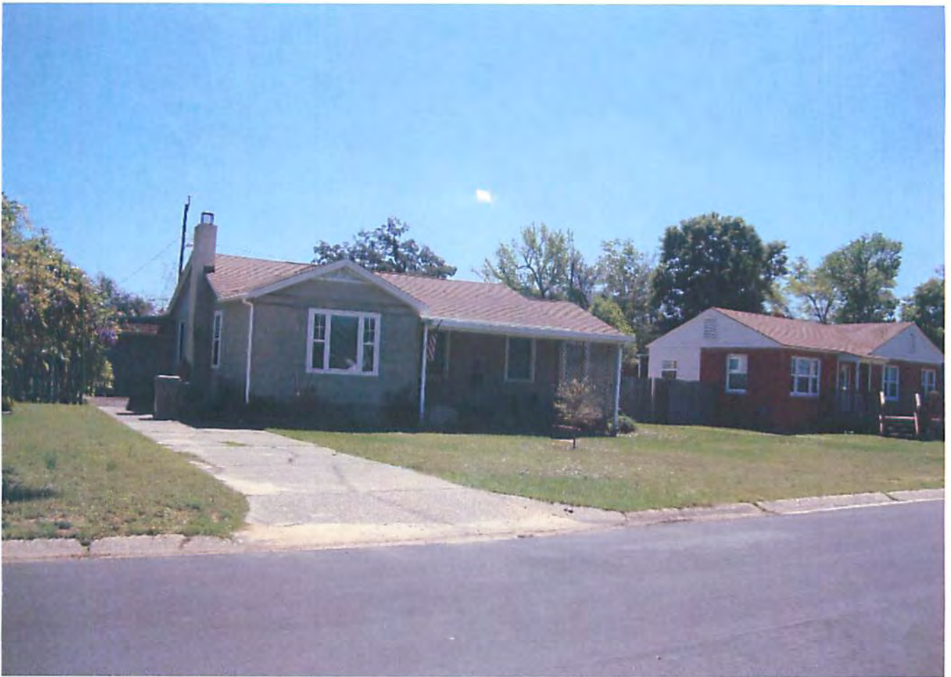
Sanitary Sewer Connections 304 Southeast Kalash Road
